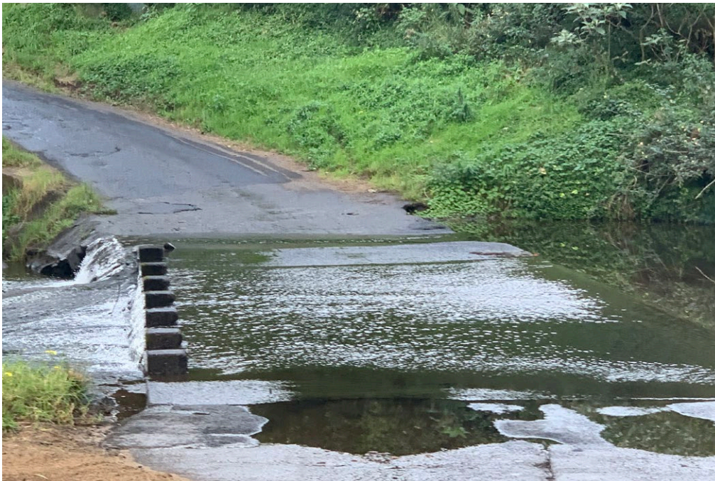
Causeway crossing of Macquarie Rivulet
