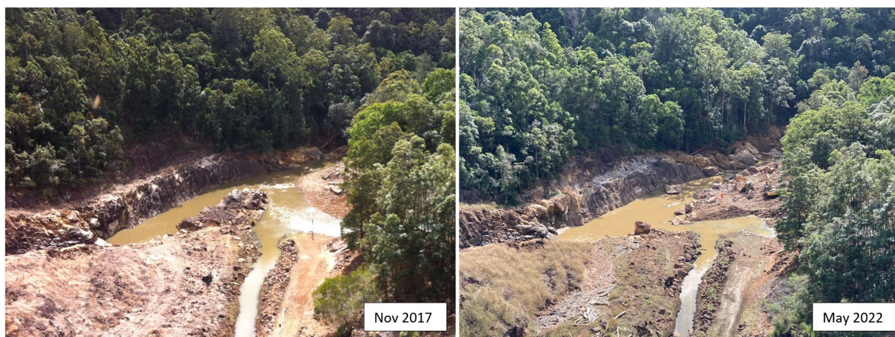
Figure 4 Spillway Erosion Pre and Post Feb 2022 Flood Event
